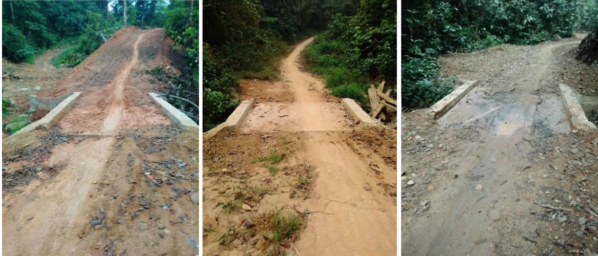
Three new box culverts constructed along Butatong-Okwangwo road with support from WCS
